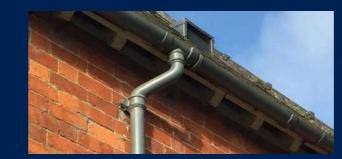
4½" Half Round Cast Iron Gutters with 2½" Round Cast Iron Downpipes
