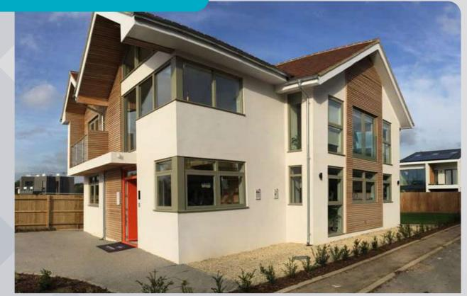
115mm Half-Round, Gutters with 80mm Round Downpipes
