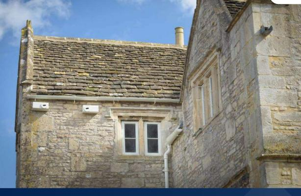
41/2" Cast iron Half Round Gutters with 3" Round Downpipes
