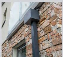
**Box Gutter and** Square Downpipes, Aluminium Canopy, Coping
