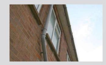
5×4" Moulded Ogee Cast Aluminium Guttering system
