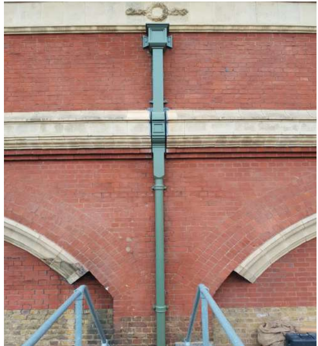
(Image) Pipe drop number thirty installed
