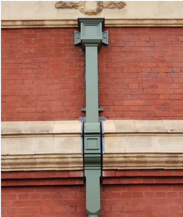
(Image) Sand Cast Moulded sections installed
