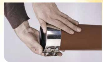
2. Ease-in one side (next to the continuity spur) then push on the opposite side of the coupling to fully seat, ensuring that the central inner register is abutted against the spigot end.
