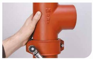
5. Check the alignment of the assembly before tightening the bolts. Alternately, tighten the bolts to ensure that the coupling is aligned evenly. Bolts should be tightened until a reasonable resistance is achieved - recommended torque setting 22 Nm.
