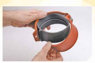
1. Slacken the bolts on the Ductile Iron coupling, fully removing one bolt completely. Remove the EPDM rubber gasket.
