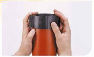
2. Push the EPDM rubber gasket over the end of the pipe or fitting, ensuring that the central inner register is abutted against the
