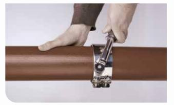
4. Evenly tighten the bolts to the required torque setting. The coupling should only be tightened once, because it cannot be dismantled and re-used. (See Couplings Data page 55)
