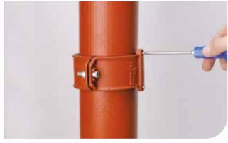
6. For electrical continuity, hand-tighten the electrical continuity screws on both sides. Ensure screws pierce external coating of pipe when tightened. (See page 55)
