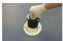
Lift out Trap using cross bar and rinse thoroughly.
