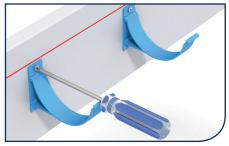
2) Using a string or laser to establish a true line and level of the gutter. Prepare to use packing pieces under brackets where there are depressions. Position fascia brackets at 900mm centres in accordance with BS EN 12056-3:2000. Fix brackets with two No 12 x 38mm round-head screws.
